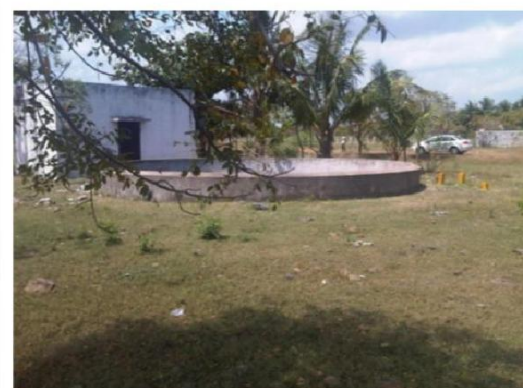
View from the eastern boundary
