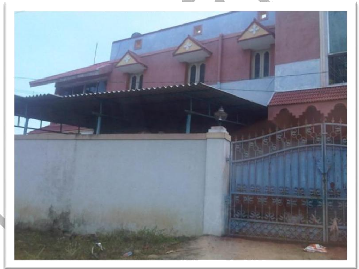
A newly built house against the main entrance of the gated community
